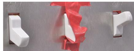
Figure 6. Taped-over light switch
